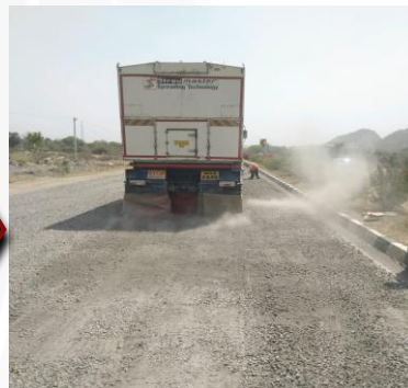
Spreading of Cement with Streu Master
