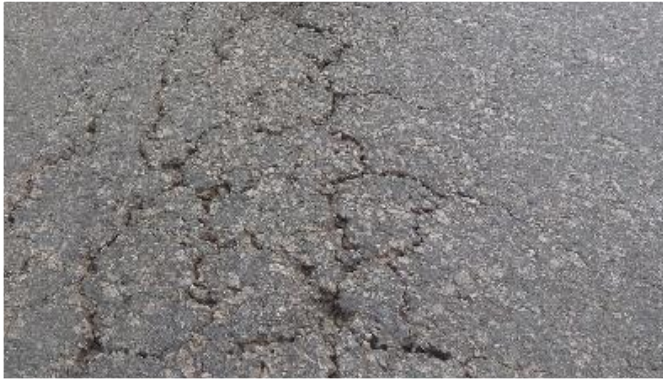
Alligator Cracks
