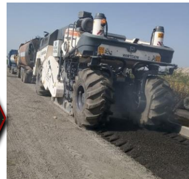
Milling & pulverisation by WR240 Wirtgen Recycler
